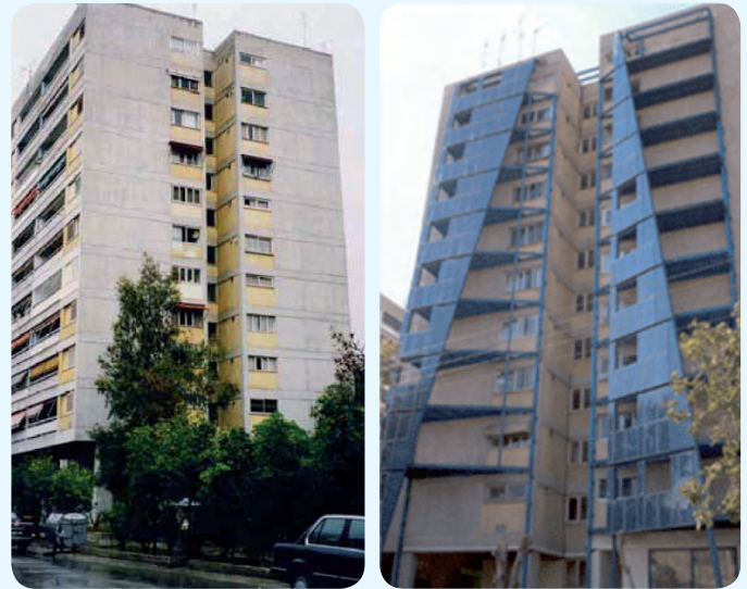
Renovation of the façade of multifamily dwellings integrating photovoltaics (Tavros, Atenas) Source: SOURSOS
